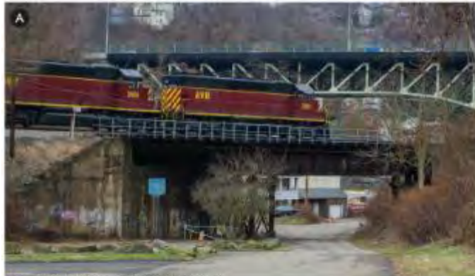
Railroad bridge over Boundary Street, entry to parking lot
